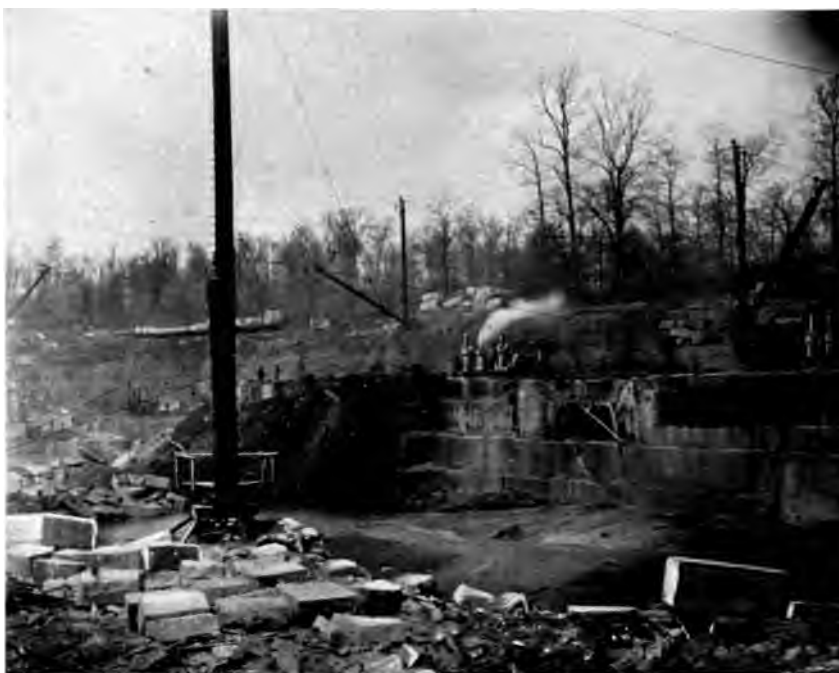
SAWING MONOLITHS FROM THE SOLID ROCK AT BEDFORD. On the Monon Route.
